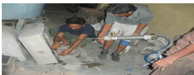
Fig . 1 Injection grouting in a slab
